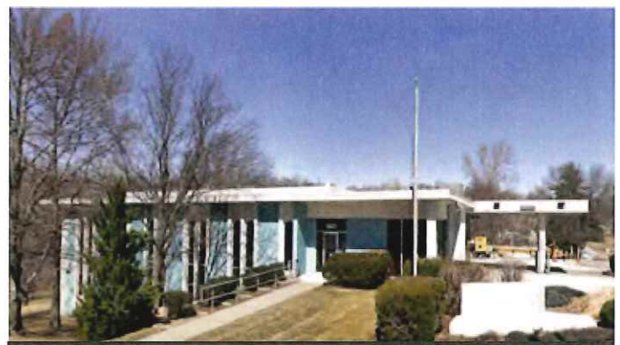
City of Independence Water Department Building built in 1964
