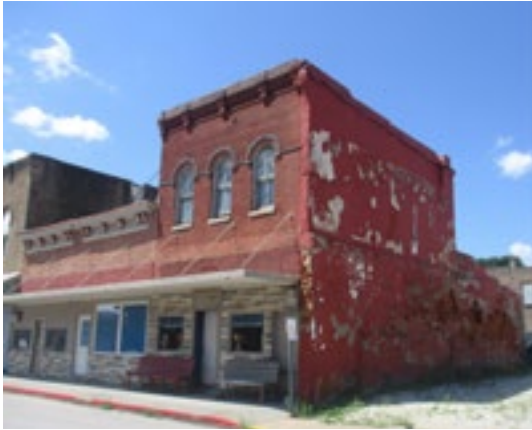
THE FORMER STONNER MEAT MARKET Chamois | Osage County
