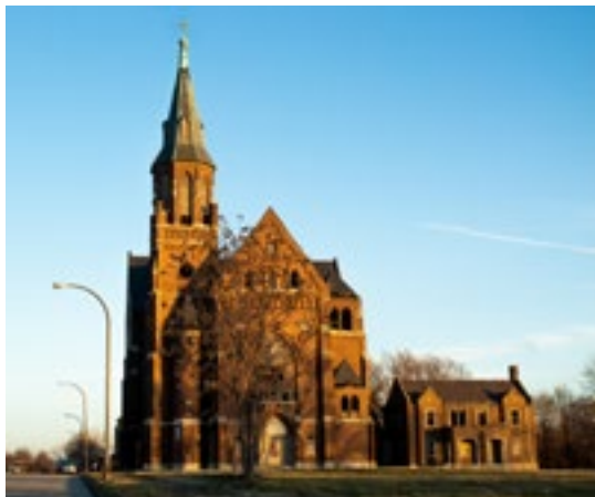
FORMER ST. AUGUSTINE CATHOLIC CHURCH "PROJECT AUGUSTINE" St. Louis City
