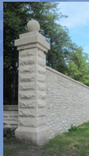
McReynolds Award MISSOURI BOTANICAL GARDEN STONE WALL RESTORATION St. Louis City
