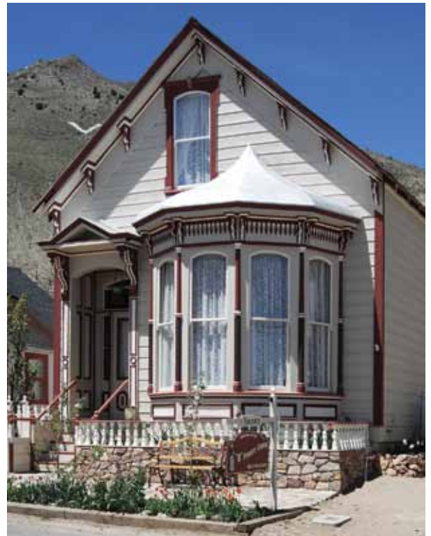
58 B Street, Virginia City, Nevada (1875). Rehabilitated as a bed and breakfast. Courtesy Chris Eichin.
