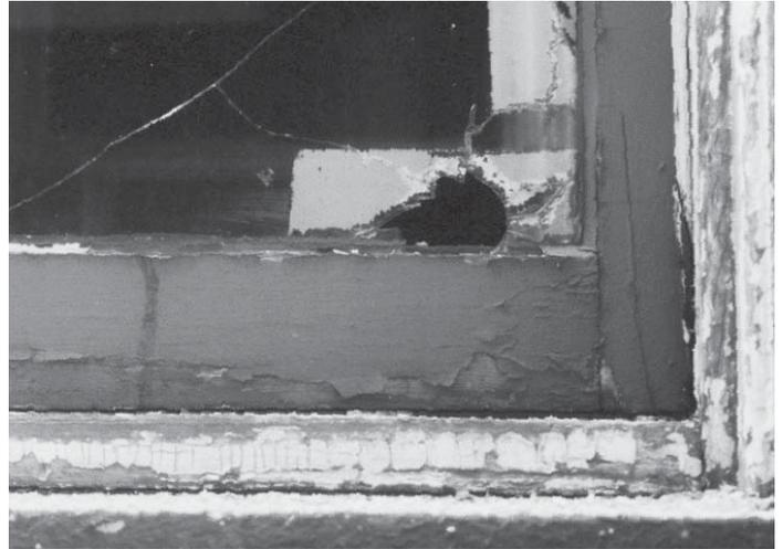
This is the bottom right corner of a window unit. The glass is in need of replacement, window and frame and sash in need of repainting, the sill and brick molding require caulking. Interior inspection reveals missing sash locks and metal spring weatherstrip needed. This window was repaired and the opening fitted with a painted metal storm window.
