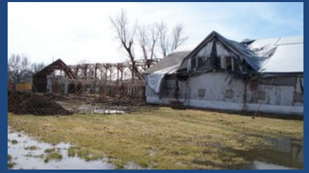
Simmons Stable undergoing renovation in 2009
